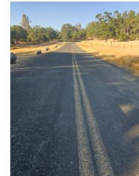
East Highland Rd. with double-yellow centerline marking
