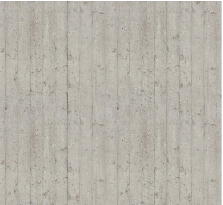
BOARD FORM CONCRETE
