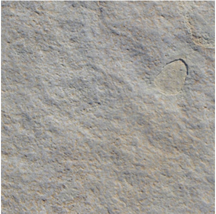
EXTERIOR STONE SURFACE
