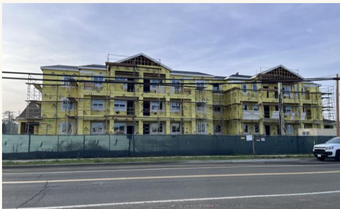
Construction activity can be a temporary source of noise.
