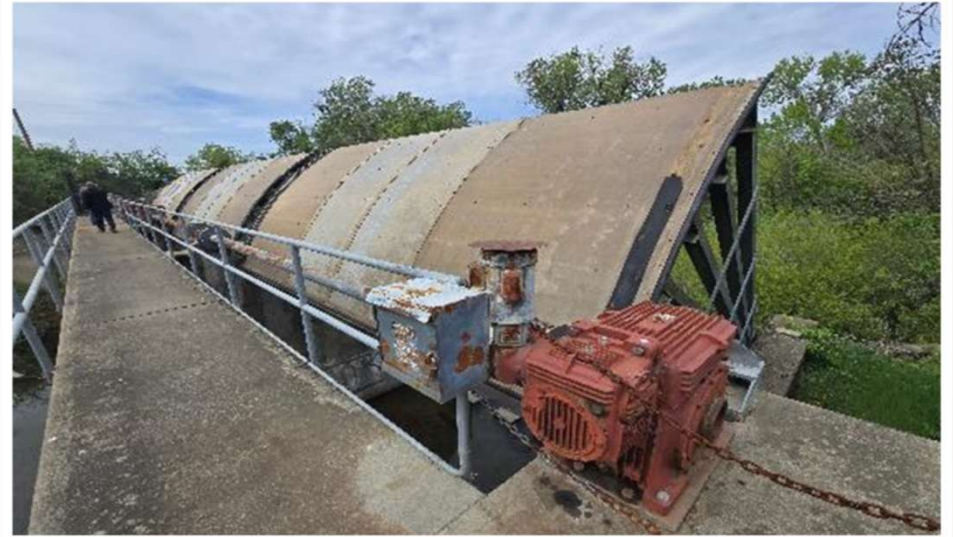
Kelsey Creek Detention Structure
