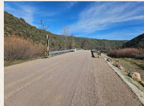
Bartlett Springs Road Bridge
