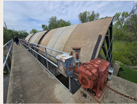
Kelsey Creek Detention Structure
