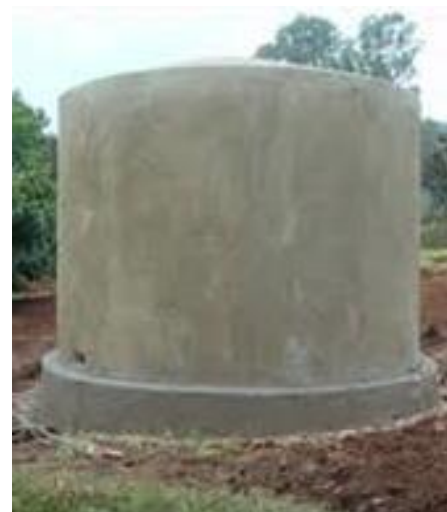
Concrete Water Tank
